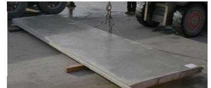
200mm of skid remaining on groove side
