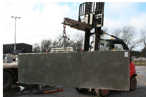
Panel being lifted from Horizontal to vertical position
