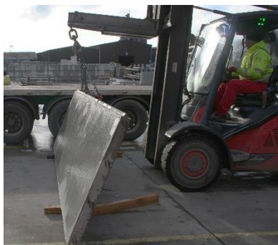
Panel being lifted from Horizontal to vertical position
