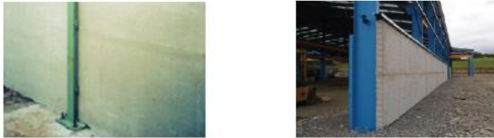
2. Slotted in between. 3. Bolted to outside face.
