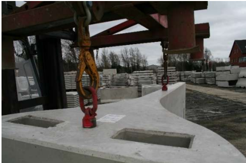
Figure 1 Swivel Eyes, Hook & Spreader Beam
