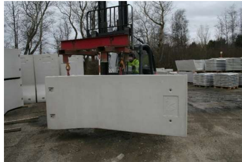
Figure 2 Swivel Eyes, Hook & Spreader Beam
