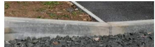
Left Hand Side Drop Kerb
