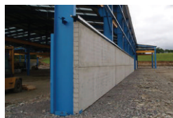
3. Bolted to outside face.
