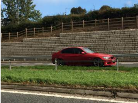
Fast construction minimises disruption to keep traffic flowing
