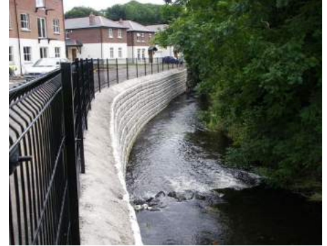
Reinforced to withstand heavy storms, these blocks can protect river banks from overflow and erosion
