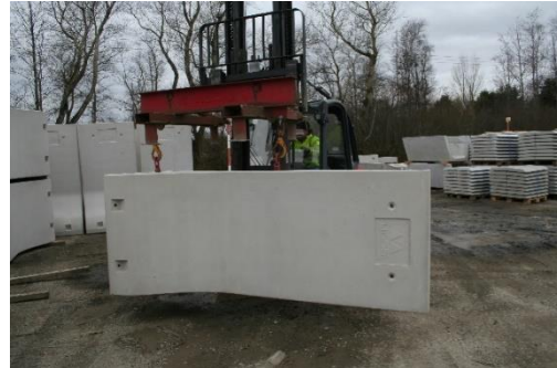
Figure 2 Swivel Eyes, Hook & Spreader Beam
