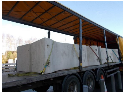
3.0m Bunker Walls being transported on their side
