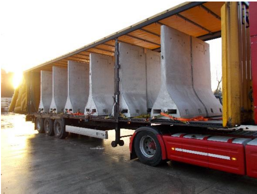
2.4m Bunker Walls being transported in their upright position
