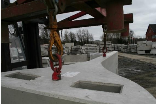
Figure 1 Swivel Eyes, Hook & Spreader Beam
