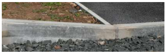
Left Hand Side Drop Kerb
