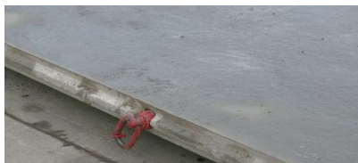
Swivel Eye screwed into Panel
