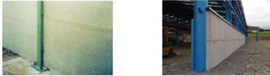
2. Slotted in between. 3. Bolted to outside face.
