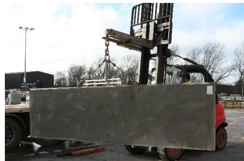
Figure 2. Panel being lifted from Horizontal to vertical position
