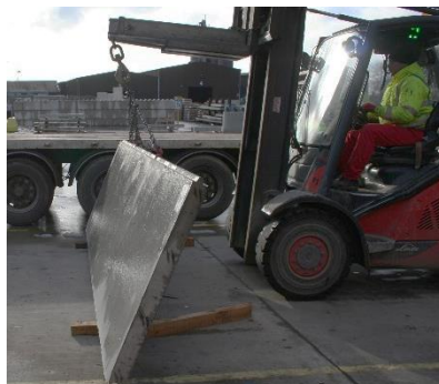
Figure 2. Panel being lifted from Horizontal to vertical position
