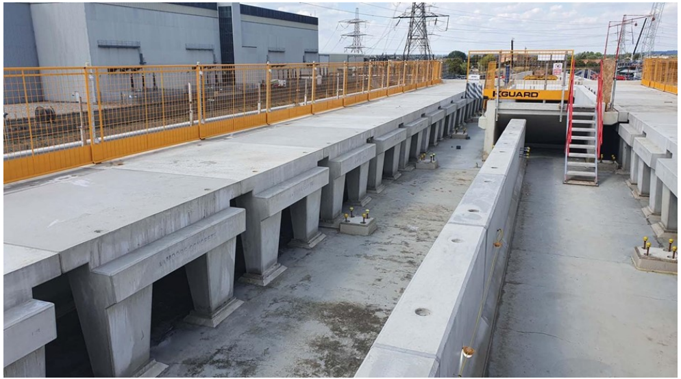
Fig1. Table units during installed on site in Barking Riverside
