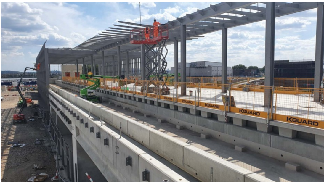
Fig2. Structural steel erection of the main platform canopy; fixed and surrounding precast concrete edge beams units, robust kerb units and table units.
