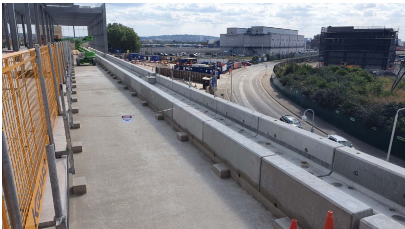
Figs4-7. Installation works from the station platform to the adjoining viaduct including Parapets & Edge Beams .
