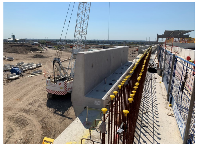
Figs4-7. Installation works from the station platform to the adjoining viaduct including Parapets & Edge Beams .
