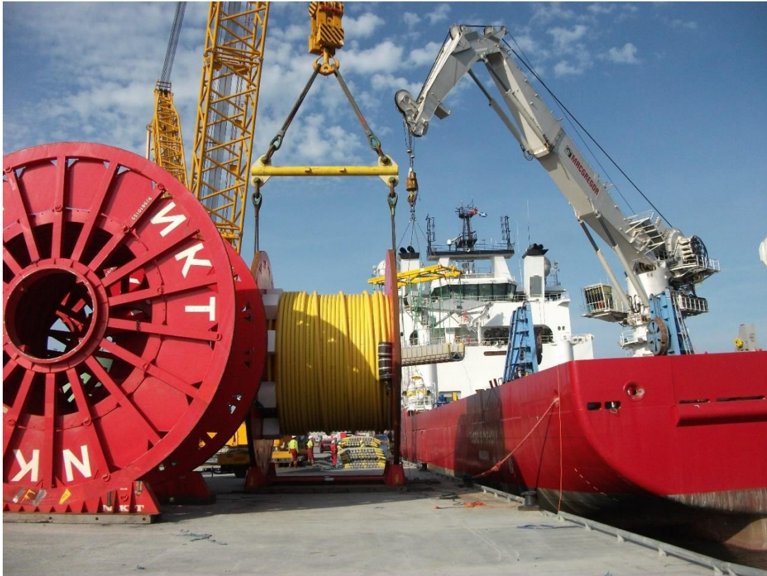
Figure 1 Moore Concrete Precast off loaded at Lerwick Harbour
