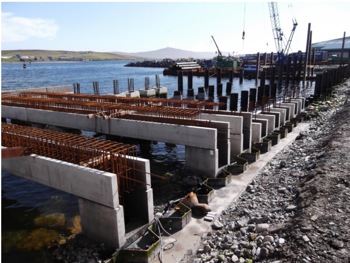
Figure 2 Moore Concrete precast unit showing the interaction between protruding steel and the in-situ steel cages.
