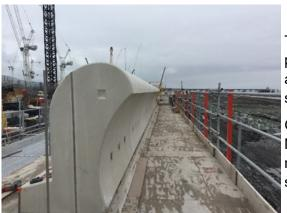
The specification of the sea wall required for the units when placed on site to be suitable to protect the nuclear facility against a 1 in 10,000-year natural hazard, such as tides, storm surges and tsunami as isolated or in-combination event.
