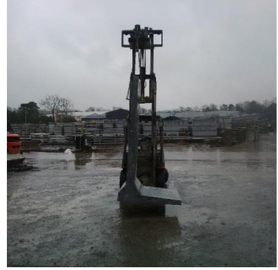
Ready for Installation
